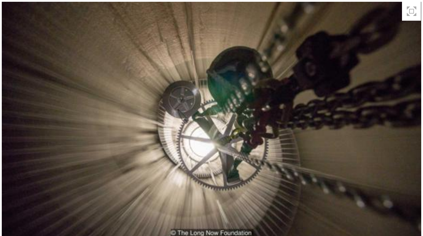
Parts of the 10,000 Year Clock being installed (Credit: The Long Now Foundation)
